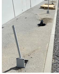
Including an EV Supply Pit during planning means in the future an electrician can simply run cable in the existing duct and terminate to a pedestal that bolts into place without additional preparation work saving precious time, money and more important to some - the need to open and reinstate pavement already in place.
